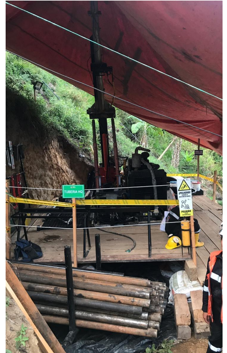
Drill Platform and rig at Chuscal 30 th September 2019
